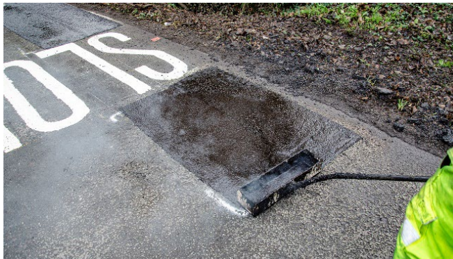
Above | Final pass of TexBand over a large pothole
