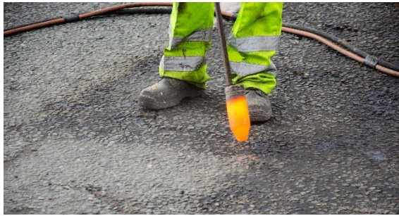
Above | Preparing the road surface with a HCA Lance
