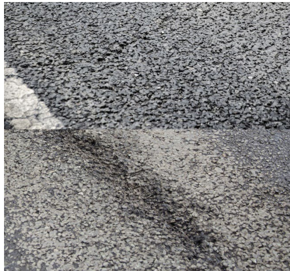
Above | Images of the smaller developing road surface cracks that TexBand would be used to prevent further deterioration as well as some of the larger surface cracks that would be repaired using TexBand.
