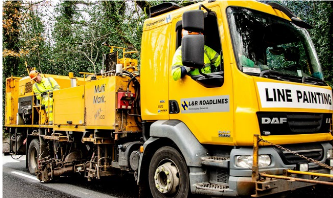
Above | L&R Roadlines crew in action installing centre lines.
