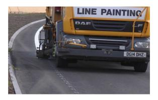
All materials are manufactured in-house by Hitex Traffic Safety. They include Hitex BBA/HAPAS Type 1 High Friction Surfacing and Hitex RainSafe road marking material, a modified performance thermoplastic that improves water drainage and reflects more light from vehicle headlights giving drivers an enhanced navigational aid to increase safety in wet conditions.
